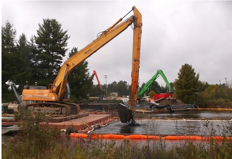
Dredging in OU1.
