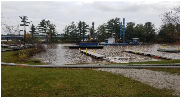
Sand and activated carbon cover placement in OU1.
