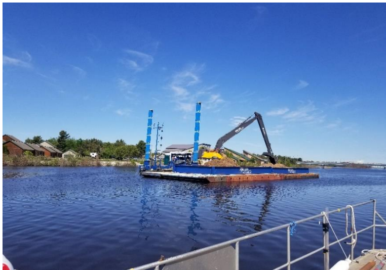
Dredging in OU2.
