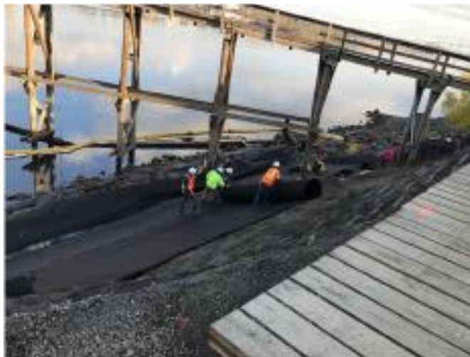
Unrolling the oleophilic biobarrier geocomposite during Phase 1 of cap construction.
