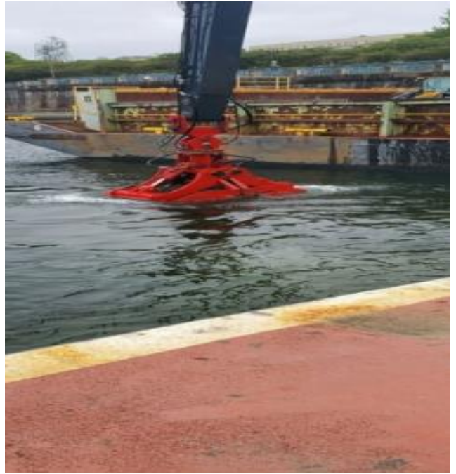
Cap material placement.
