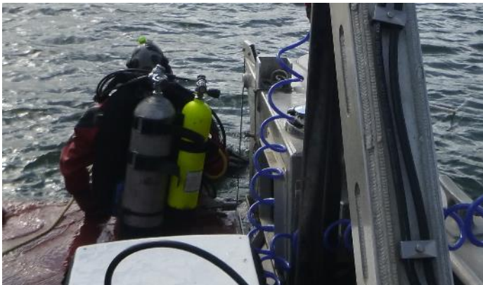
Diver Assistance during Sampling Port Installation.
