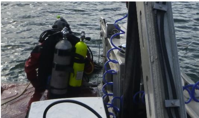
Diver Assistance during Sampling Port Installation.
