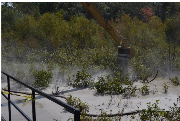
Amendment placement in the Heavily Vegetated Area.
