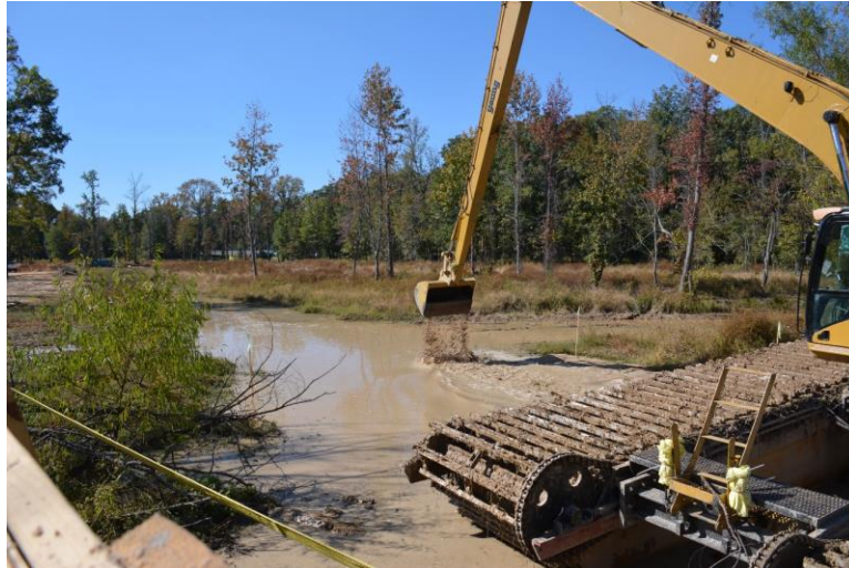
Reactive cap placement in the Open Water Area.
