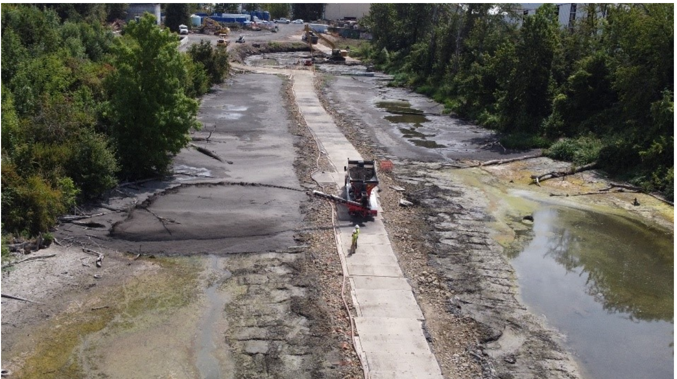
Figure 6-4. Conveyed aggregate delivery.
