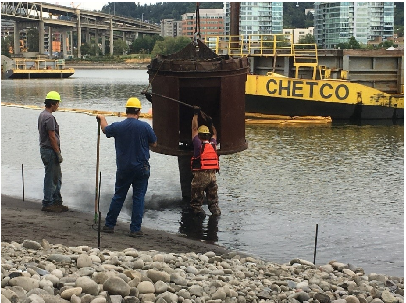
Figure 6-6. Aggregate hopper.
