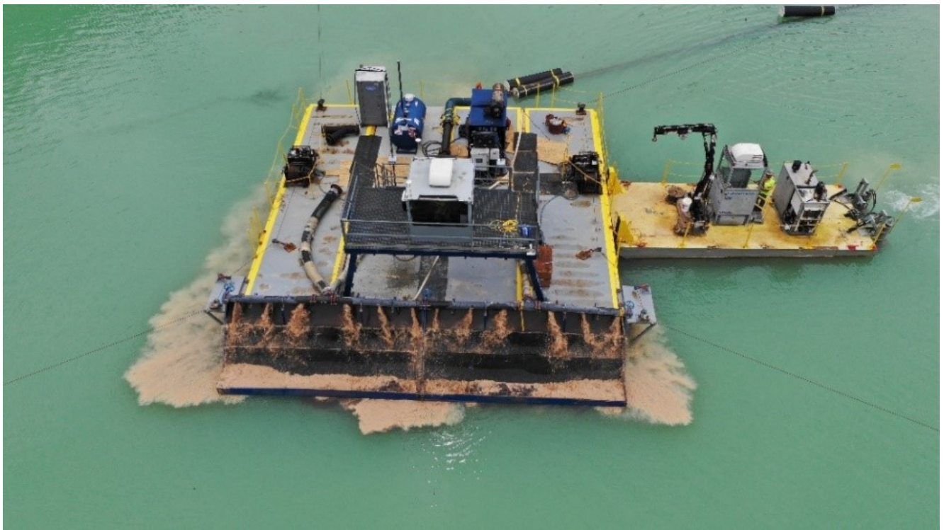
Figure 6-8. Hydraulic capping system.
